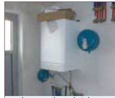
condenserende gasketel (rendement 109%)
